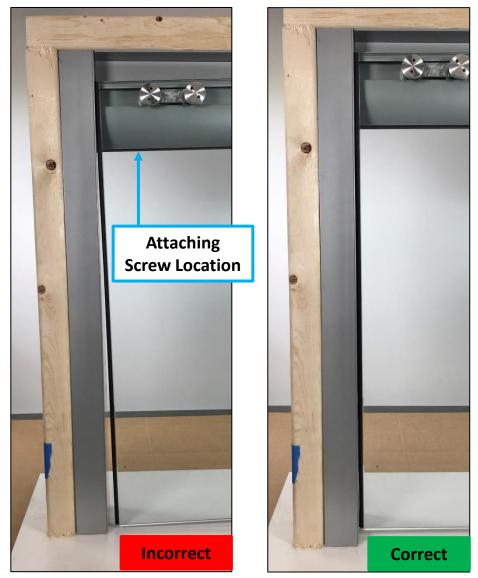
If there is an uneven gap between the framing and the door when the door is closed, adjust the attaching screw within the door opening to create tight and even gap.
