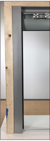
Install the D-Pad on the edge of the door. The D-Pad will close any light gap between the framing and the door when the door is closed.
