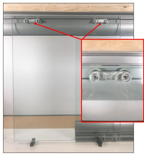
With the Carriages already in the View Track, place the glass door on shims to align the holes in the door with the Carriages. Press the door tight to the View Track to allow the Carriages to go through the holes, as shown above.
